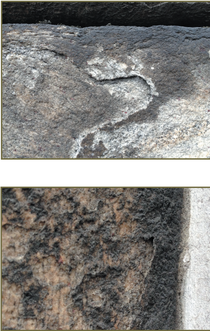
Figure 8. Degradation observed in historical buildings and identified as black crust. Formed by the accumulation of particles deposited on the flat surface of fine-grained garnet gneiss, the crust is associated with a blistering process on the façade of the Carmelite church, Rio de Janeiro.
