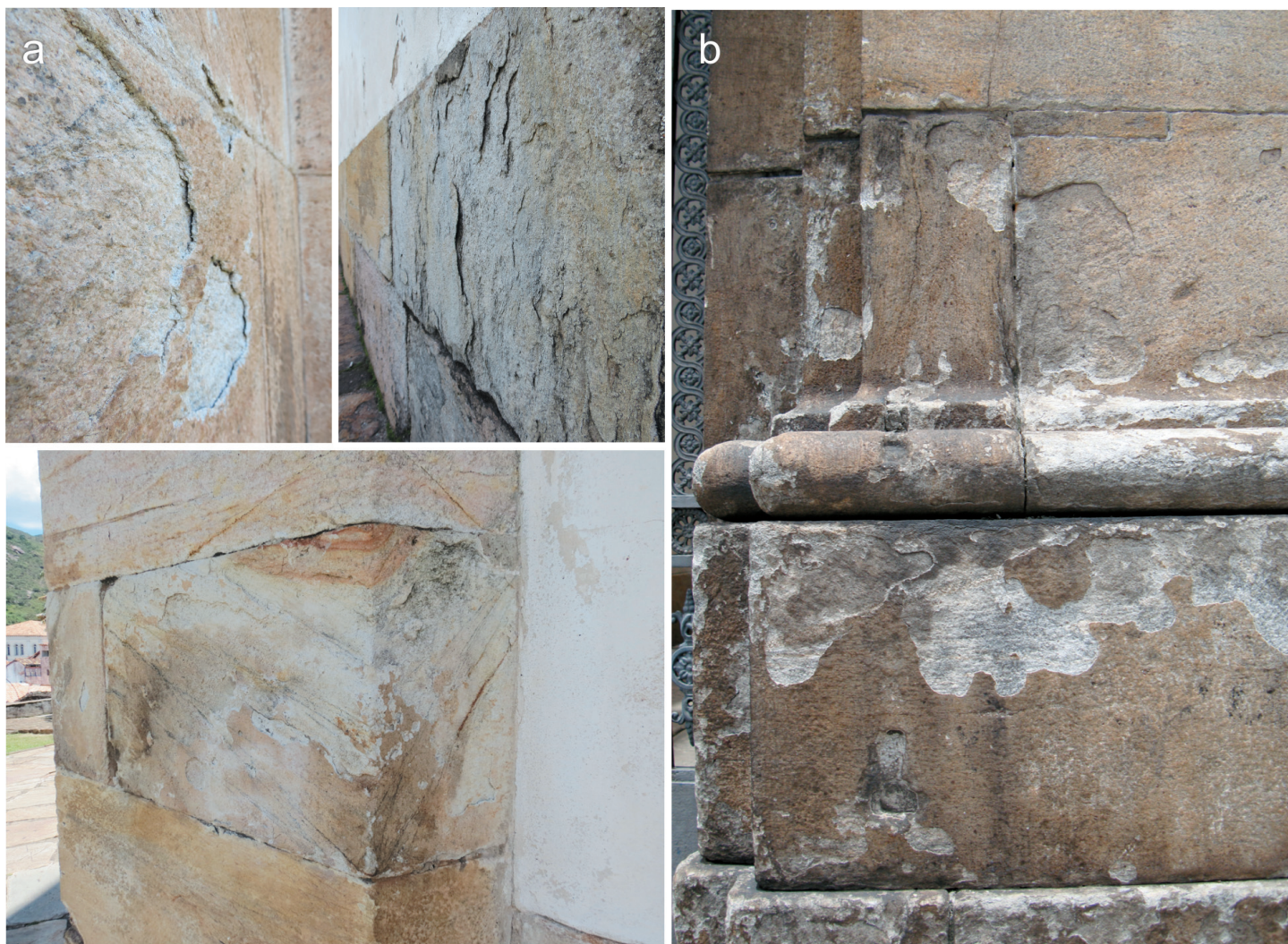
Figure 5. Example of stone detachment as flakes or scales (spalling). In this case, detachment is parallel to the block surface but not to the rock structure, as observed in a) the external and flat wedges of quartzite at the Carmelite Chapelin, Ouro Preto, Minas Gerais, and b) gneiss at the Carmelite Church in Rio de Janeiro.
