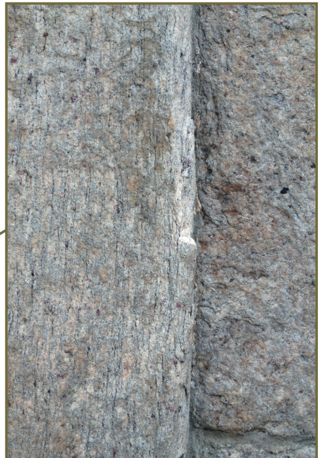
Figure 4. Detachment processes observed in parallel-cut blocks in which surface exfoliation is parallel to vertical foliation planes (schistosity) in a) a sericite-quartzite application in Ouro Preto, Minas Gerais, and b) a garnet gneiss application in the city of Rio de Janeiro.
