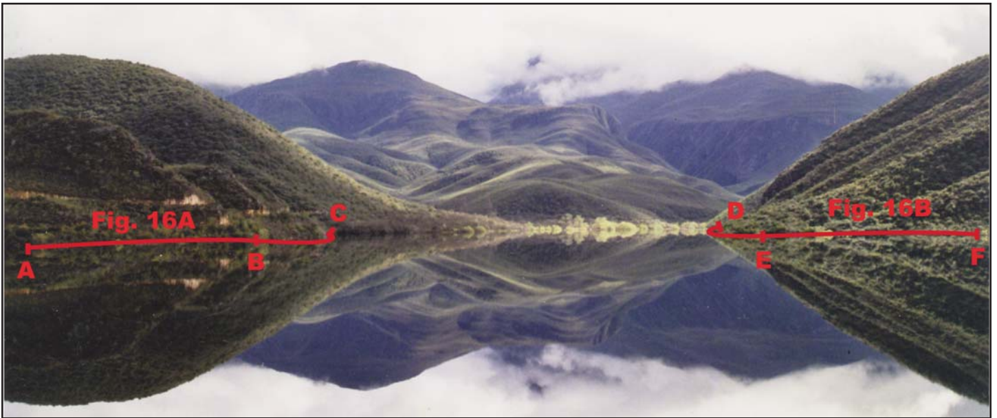
Figure 15. General north-facing view across the lake of Koos Raubenheimer Dam (Section 4, Map 1), showing the location of detailed cross-sections along the western and eastern banks in Figures 16A and 16B, respectively.
