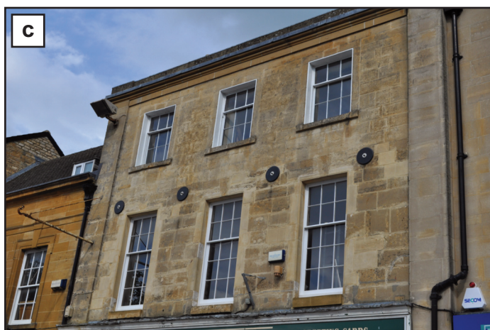
Figure 4. Examples of controversial or poor practices of stone usage. a) Queen Elizabeth II Courtyard, British Museum, London; b) contrasting replacement of stone in the interior of the Lincoln Cathedral, and c) replacement with stone of a different colour disrupting the original colour pattern in the exterior of the cathedral, Chipping Norton, Oxfordshire.
