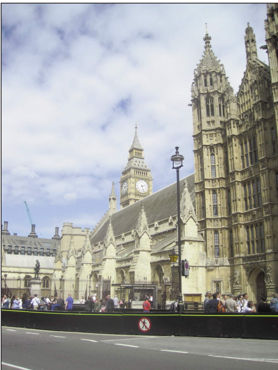
Figure 2. The Palace of Westminster showing pale-coloured Clipsham Stone from recent repairs, contrasting with Clipsham Stone from previous repairs and Anston Stone.
