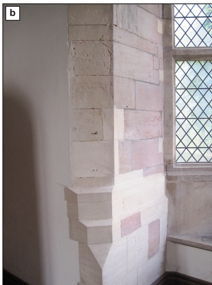
Figure 4. Examples of controversial or poor practices of stone usage. a) Queen Elizabeth II Courtyard, British Museum, London; b) contrasting replacement of stone in the interior of the Lincoln Cathedral, and c) replacement with stone of a different colour disrupting the original colour pattern in the exterior of the cathedral, Chipping Norton, Oxfordshire.
